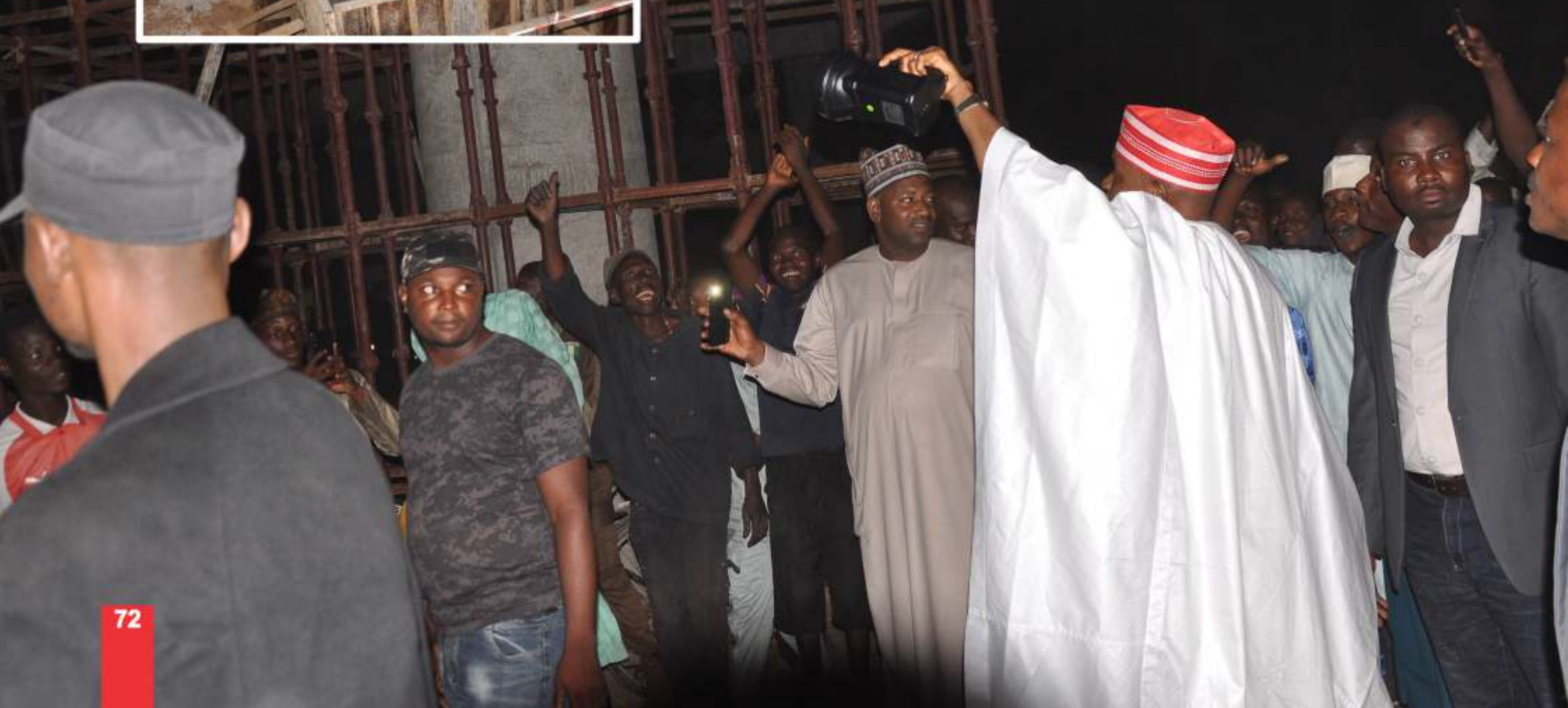
Night Visit: Ongoing Construction of Tal'udu Bridge
